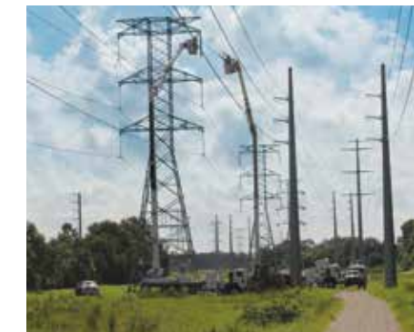
Crews upgrade large transmission lines that connect SEC to Taft.
