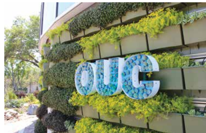
Vertical garden at Gardenia Operations Center.
