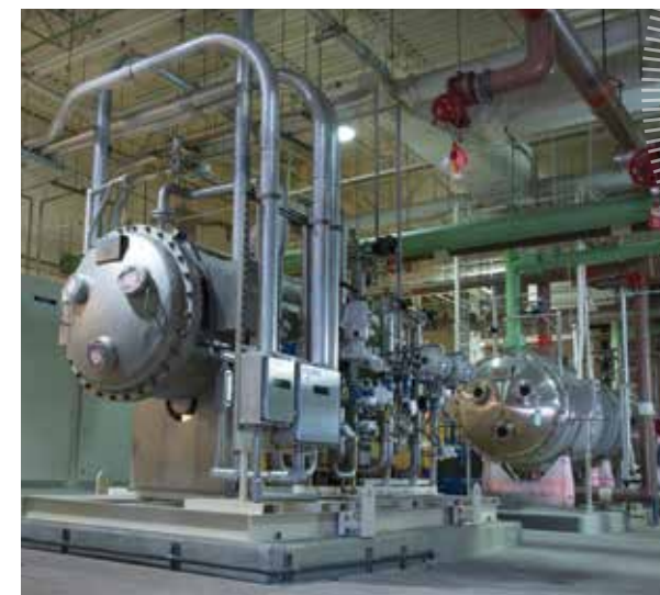
Upgraded ozone generators at the Southwest Water Treatment Plant were the first in a series of improvements to the system.
