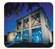
With *OUCooling*, all cooling equipment — the cooling tower, pump and chiller — is housed in one centralized, offsite location. At this facility, water is cooled to 37 degrees and pumped through underground pipe loops to participating buildings. Warm air is circulated over chilled water coils at each building, providing a steady, reliable flow of cool air. The water is then recycled to the central chiller facility to be cooled again before returning to the loop.
