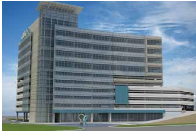
OUC's new administration building, scheduled to open in late 2008, will be the greenest building in downtown Orlando.
