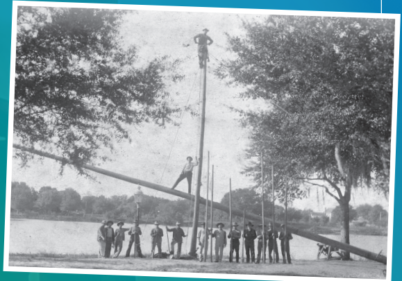
Utilities workers place Orlando's first electric pole that would serve as the foundation for the birth of OUC.
