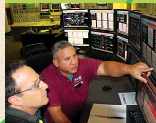
Project Engineer Eric Costello (from left) and Plant Operator Richard Zayas monitor the fuel mix inside the Stanton Energy Center Control Room.
