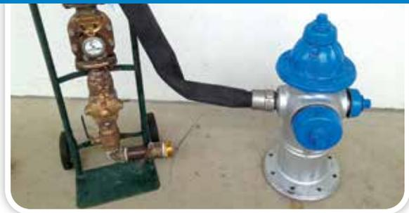
OUC portable water meters can only be utilized within the OUC water service territory. OUC water territory is defined by silver barrel (body) and blue cap painted hydrants. Secure and transport meters safely; never leave unattended. Use OUC-approved fire hydrant wrenches (available in OUC's Water Meter Shop). **FLUSH FIRE HYDRANT UNTIL WATER IS CLEAR BEFORE ATTACHING PORTABLE WATER METER.** Install assembly in vertical upright position. Operate in horizontal position (with dial facing up).
