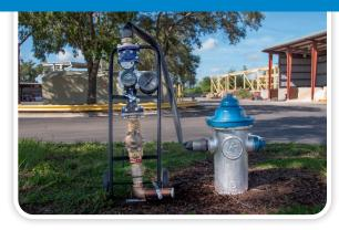
OUC portable water meters can only be utilized within the OUC water service territory. OUC water territory is defined by silver barrel (body) and blue cap painted hydrants. Secure and transport meters safely; never leave unattended. Use OUC-approved fire hydrant wrenches (available in OUC's Water Meter Shop). FLUSH FIRE HYDRANT UNTIL WATER IS CLEAR BEFORE ATTACHING PORTABLE WATER METER. Install assembly in vertical upright position. Operate in horizontal position (with dial facing up).
